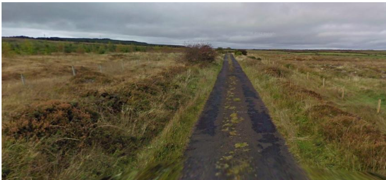
Plate 16 – Street View of Site Pinch Point 18
