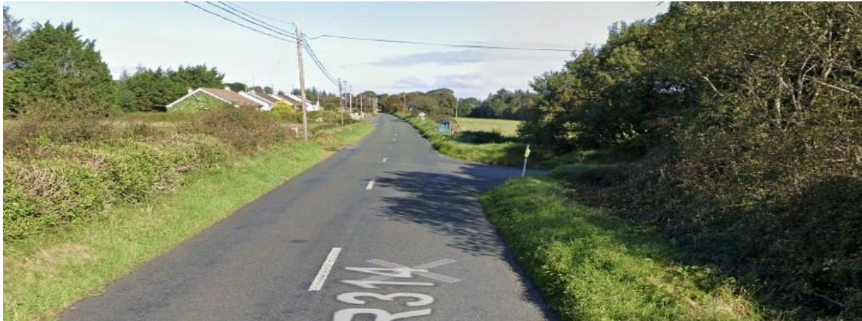
Plate 20 – Street View of Pinch Point 15
