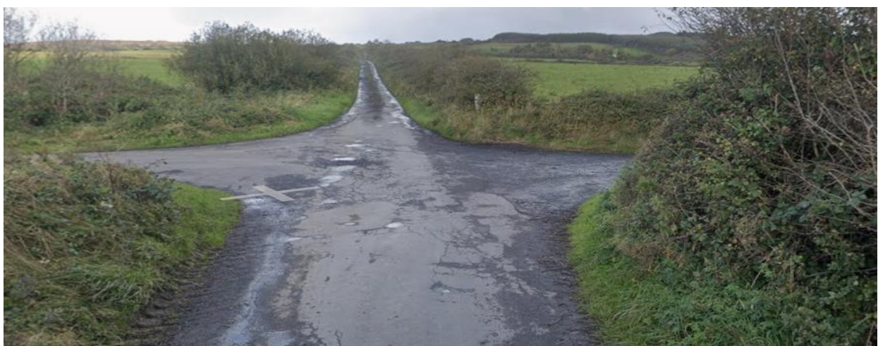
Plate 9 – Street View of Pinch Point 9
