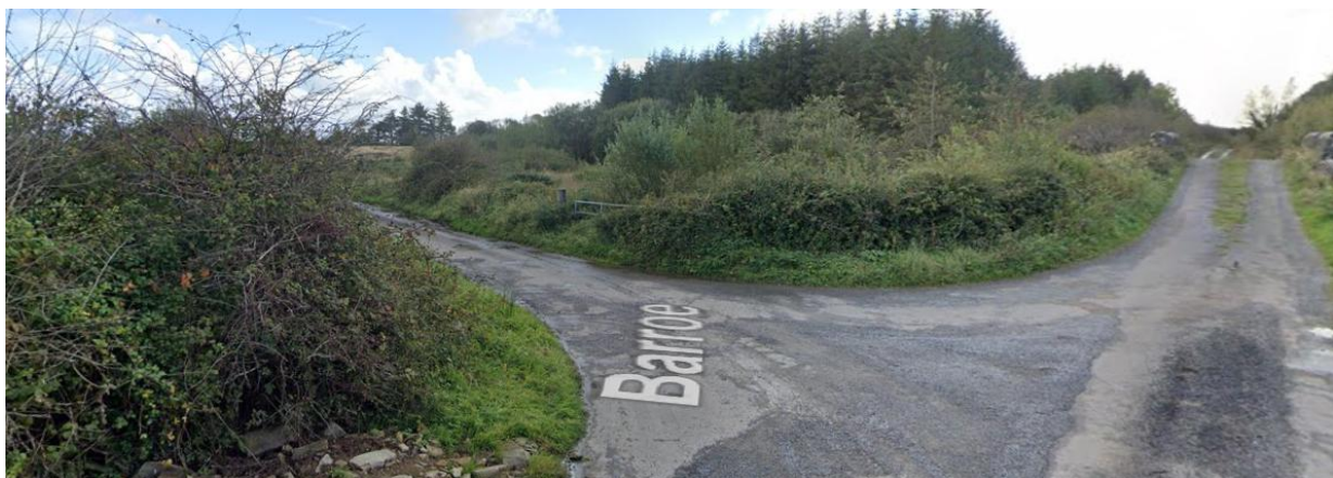
Plate 10 – Street View of Pinch Point 10
