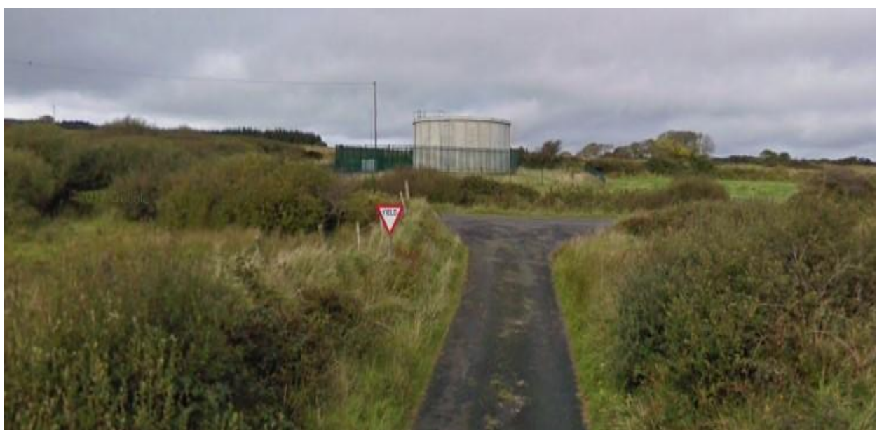
Plate 17 – Street View of Pinch Point 19
